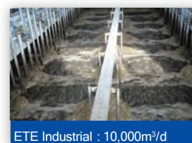
ETE Industrial : 10,000m³/d
